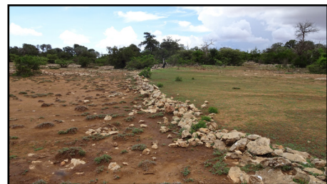
One of the many rock barriers constructed by local staff and visiting students to reduce soil erosion.
